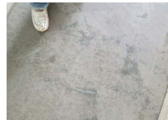
Concrete floors typically have an uneven appearance.
