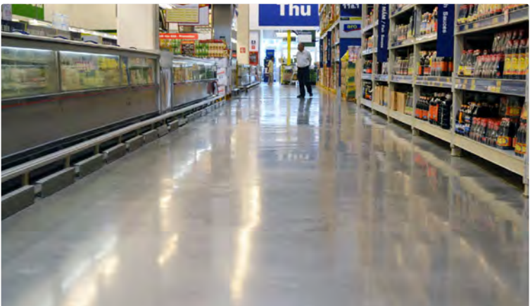
A few months after concrete densification, and with typical foot traffic and regular cleaning, a glossy sheen has naturally developed on the floor surface.
