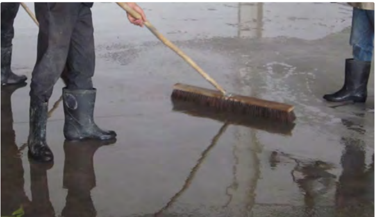
Chemical densifier is applied as a flood coat and broomed into the concrete surface allowing for complete penetration and chemical reaction.
