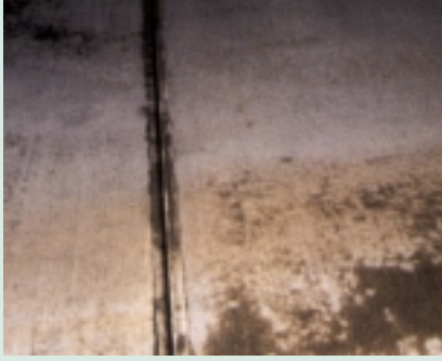
13. Over troweling can entrap moisture and create dark areas.
