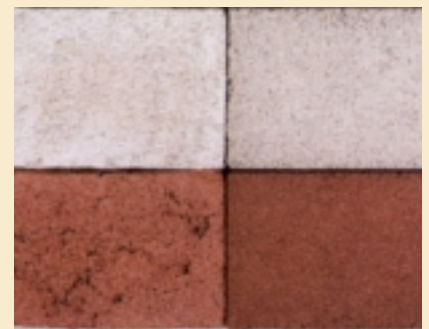
12. different water/cement ratios make plain (top) and colored concrete (bottom) appear pale or faded.
