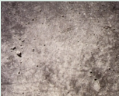
16. Excessive use of form release agents can contribute to discoloration and voids in a formed concrete surface.
