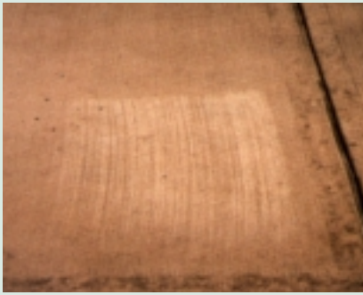
15. The pale broom mark, which is permanent, shows the first broom stroke after the broom was wetted.
