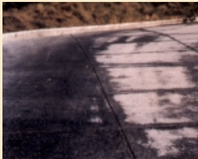
6. Carbon black pigments can leach out of concrete in wet areas unless adequately sealed.
