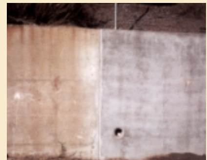
22. These stains could have been avoided by diverting runoff from the concrete face.
