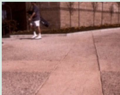
8. While exposed aggregate was used in this project as a design feature, a similar effect can occur due to wear and erosion.
