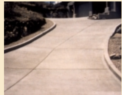
21. After curing. Concrete lightens as it cures. Most change occurs within 30 days.
