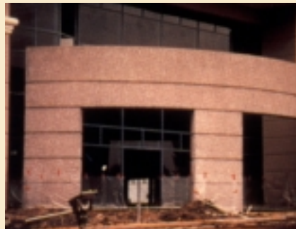
18. After sandblasting. A more uniform color was revealed after the cast-in-place wall was fully cured and sandblasted.
