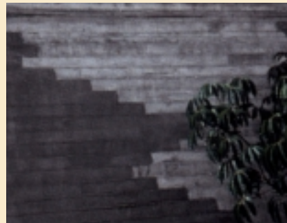
19. Variations in the porosity of lumber form work cause uneven absorption of water from the concrete, resulting in uneven color.
