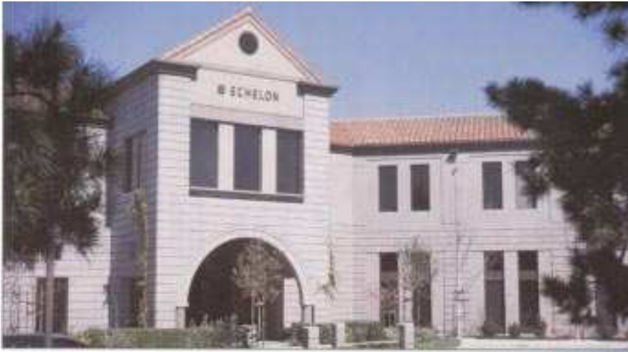
Northern California's Central Concrete applied its usual tight quality control in delivering integrally colored mixes for the Echelon Building in Pal Alto, a recent tilt-up job with general contractor Devcon. (Photo: Davis Colors)
