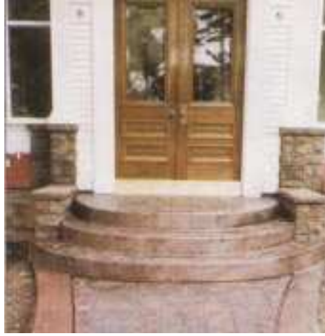
Pine Hill Concrete Mix Customer, Broad Spectrum Concrete, blends new integrally colored, patterned stamped flatwork and steps with vintage masonry.
