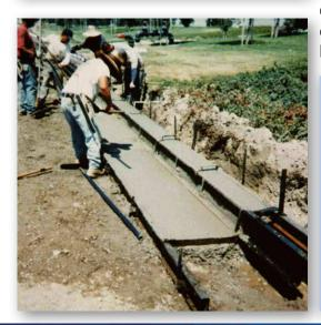
The Curb Smart forming system is versatile product that adapts to many concrete forming conditions. It is ideally suited for applications that include sidewalks, driveways, curb and gutters, pavements, footings and industrial slabs.
