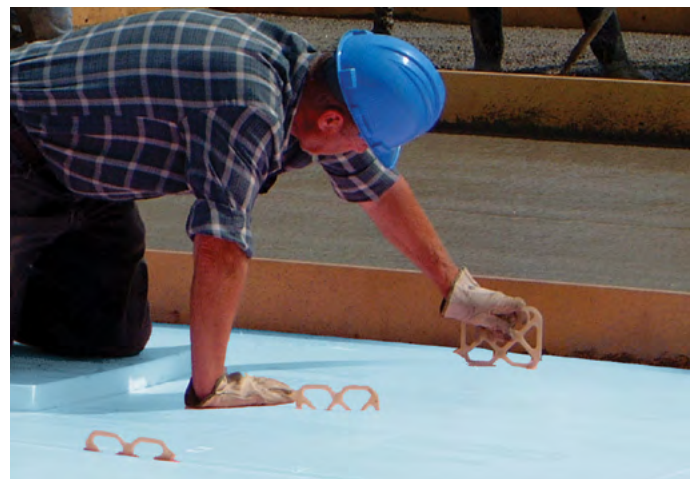
The third wythe — the interior wythe — being installed over the insulation, incorporating the Delta Tie and rebar.
