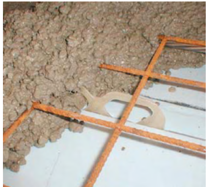
The third wythe — the interior wythe — being installed over the insulation, incorporating the Delta Tie and rebar.
