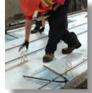
depth, move the tie slightly so that the reinforcing mesh sits in the depressed "V" section of the tie. NOTE: The minimum Delta Tie embedment into the fresh concrete is 1½".
