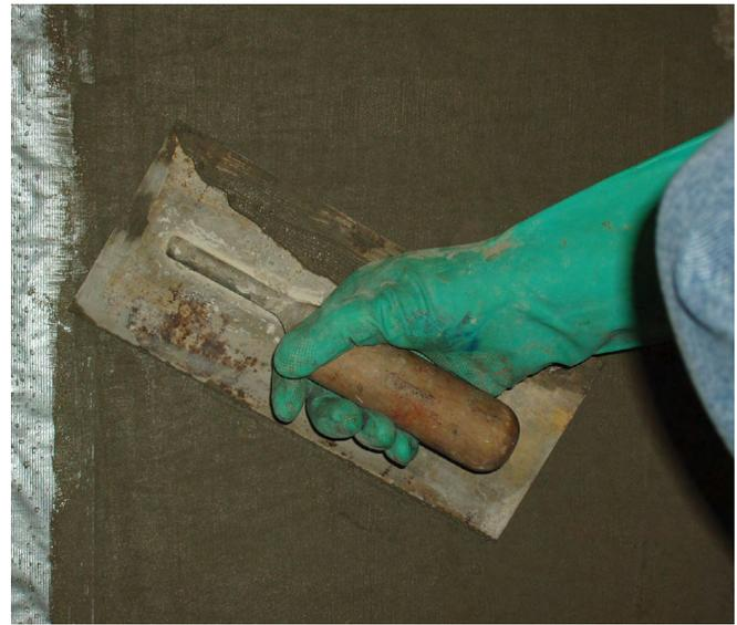
**Thin Resurfacer***Horizontal Repair Mortar*
