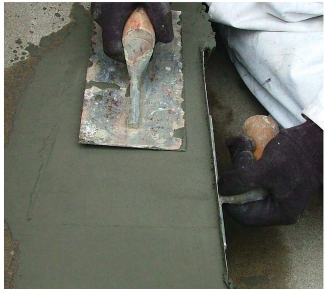
**HORIZONTAL****HD 50***Horizontal Repair Mortar*
