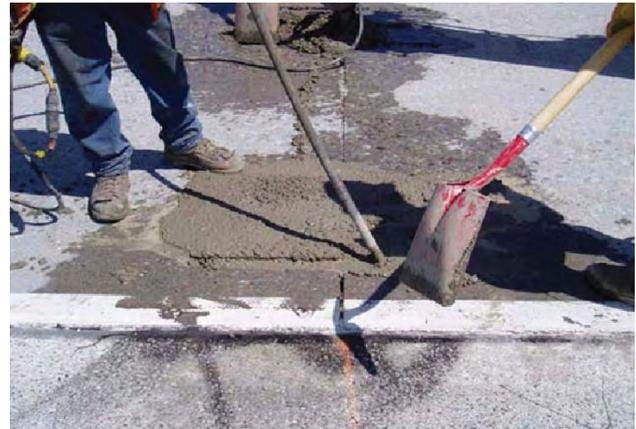
**EPOXY JOINT FILLER****Pro-Flex***Epoxy Joint Filler*
