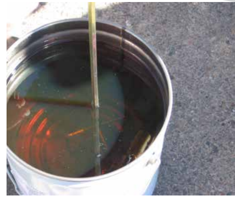
Blend epoxy components
