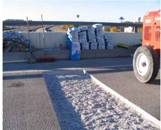
Road repair with HD 50 by Dayton Superior
