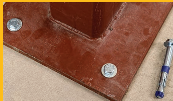
➤ Structural column connection
