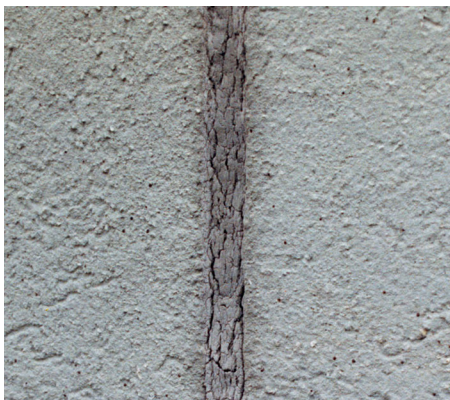
Failed urethane sealant in EIFS joint
