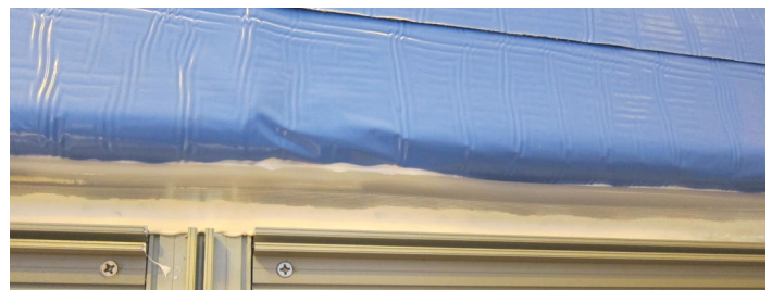
Figure 14: Finished strip installation
