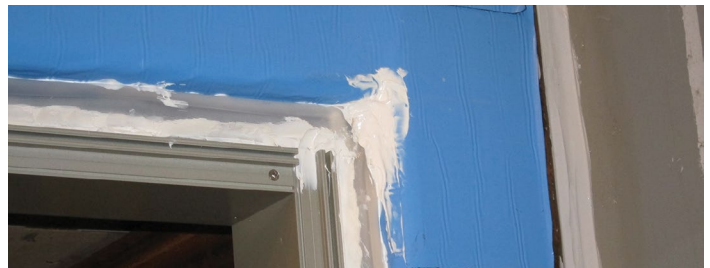
Figure 12: Folded and sealed corner
