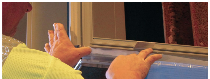
Figure 13: Folding strip onto mullion and attaching with sealant
