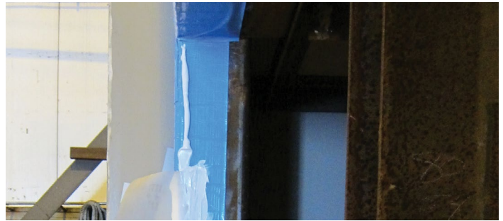
Figure 8: Keep splices a minimum of at least 12 inches (300 mm) from corner
