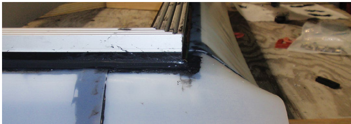
Figure 2: Corner and strip pieces installed in-shop
