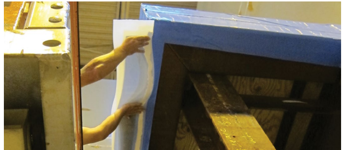
Figure 9: Installing strip at head of fenestration unit using sealant
