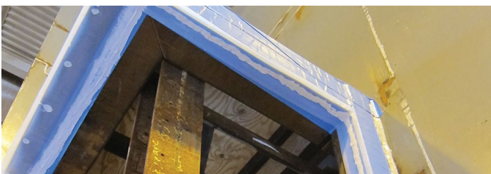
Figure 7: DOWSIL™ Silicone Transition System-wrapped opening
