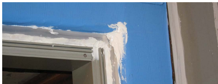
Figure 12: Folded and sealed corner
