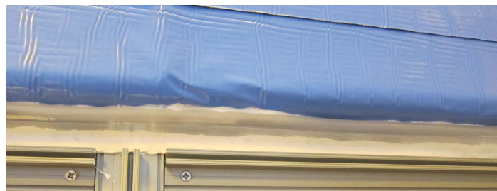
Figure 14: Finished strip installation
