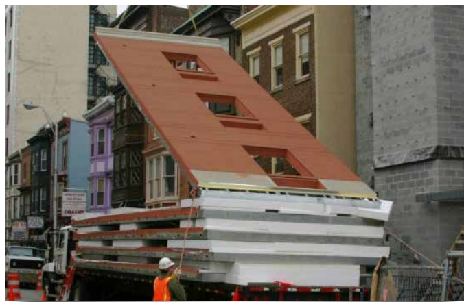
Outsulite panel installation
