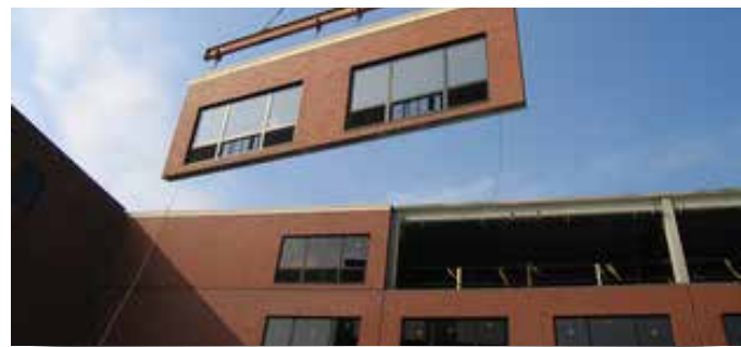
Outsulite panel installation
