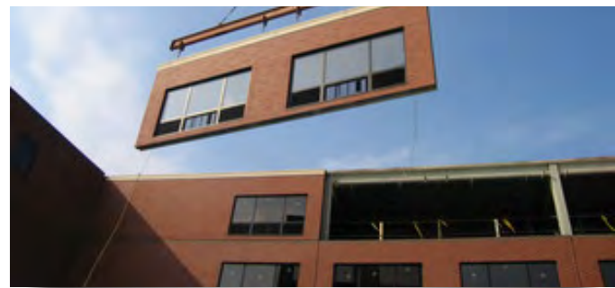
Outsulite panel installation
