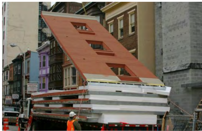
Outsulite panel installation
