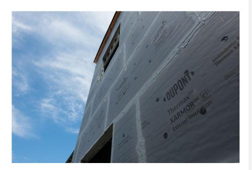
DuPont<sup>TM</sup> Thermax<sup>TM</sup> polyisocyanurate insulation products offer consistently high, long-term thermal resistance, exceptional fire protection and a wide variety of sizes and facers.
