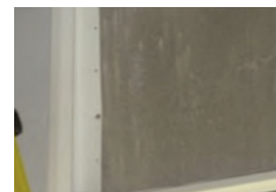
PVC attached to tilt-up wall
