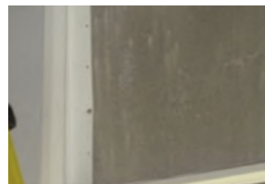
PVC attached to tilt-up wall
