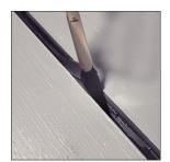
Smooth surface of silicone with caulking knive and insert end back into the joint.
