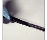
• Tool the top edge of the sealant silicone bead to a smooth blend with the outside edge of the bellows.
