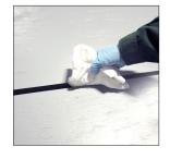
Wipe joint faces to ensure joint sides are free of dust, previous sealant, oils, grease, etc.
