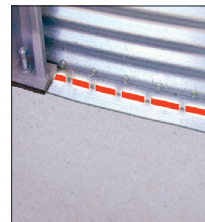
Sill Plates and ground level water seams
