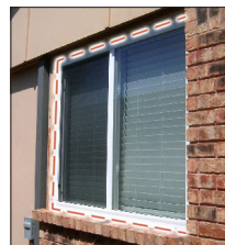
Window Casings and other finished areas
