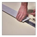
As soon as the material is placed into the gap place at least four weights\* along the length of the coverplate.
