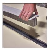
The precompressed foam will begin to expand to fill in the expansion gap.
