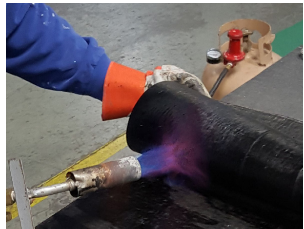
Torch applying heat to mod bit waterproofing membrane. Consult the membrane manufacturer for specific installation guidelines.
