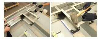
Working away from the ends of the transition, connect the straight lengths of rail and install straight lengths.
