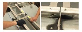
TIP – Sometimes the metal pins will not align easily. To fix this loosen the screws in the capping strips that hold the clamping spacers. This will give you some 'play' to help with pin alignment. Once aligned, retighten the screws.
