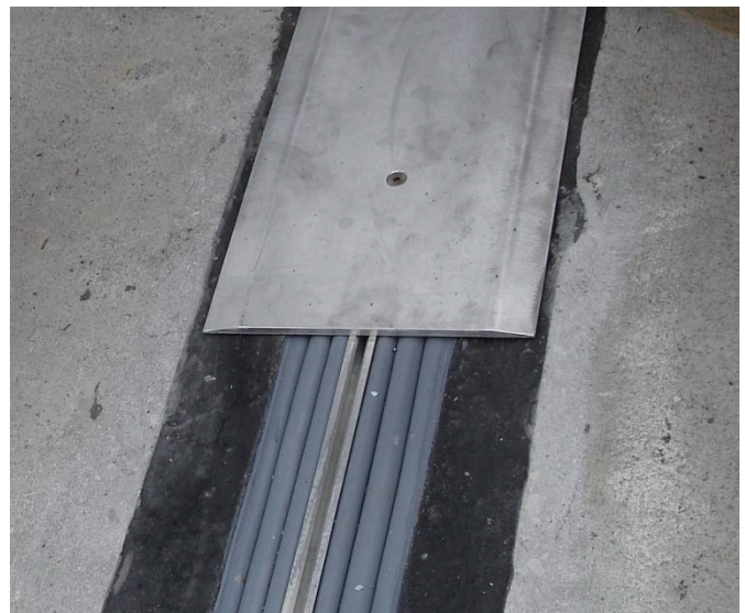
SJS-FR System installed with Emcrete elastomeric nosing material in blockouts on each side of joint gap.
