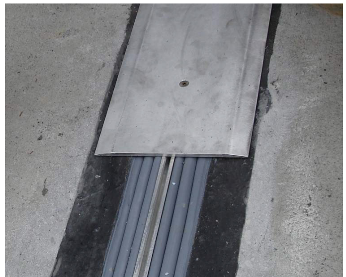
SJS System installed with Emcrete elastomeric nosing material in blockouts on each side of joint gap.
