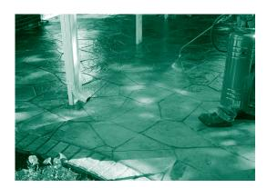
When spraying, the product should exit the nozzle in a fine and even fan pattern. If there are streams of material coming out of the nozzle, the sprayer either needs to be pumped up with more pressure, or a nozzle with a larger orifice size should be used. Most sprayers come equipped with a 0.5 gallon per minute (1.9 liters per minute) spray nozzle, but for higher solids materials, a 1 gallon per minute (3.8 liters per minute) nozzle may be required to produce an even spray pattern.
