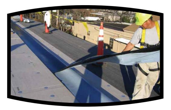
The top of the BASEGARD SA sheet is sand surfaced to provide a suitable substrate for heat welding, hot asphalt, and insulation adhesive attachment methods. The bottom surface has an opaque split release film for easy installation.
