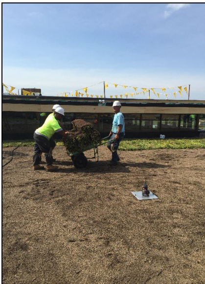
Rolled Sedum Mats being staged at the jobsite.
