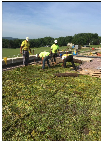
Sedum Mats being installed at the jobsite.
