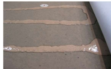
Close up of 12" Bead Spacing
