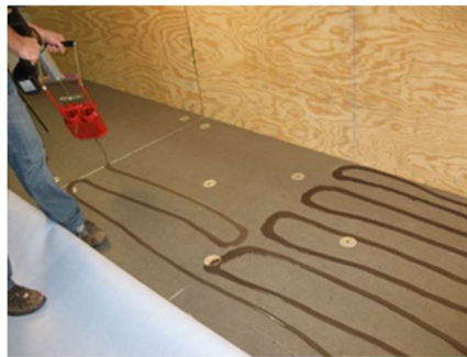
Bead application of XR Stick in cartridge on mechanically attached Polyisocyanurate insulation board @ 6" o.c.
