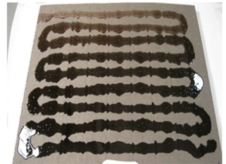
Freshly applied beads of XR Stick on mechanically attached Polyisocyanurate insulation board @ 4" o.c.
