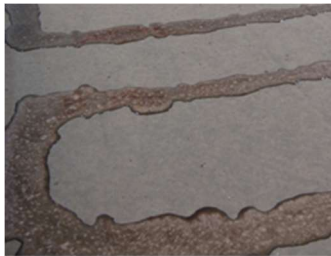
STEP 1: Freshly applied ISO Spray R Adhesive / XR Stick - cream stage
