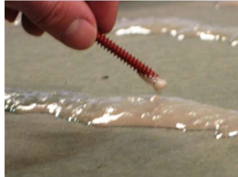
STEP 2: Allow ISO Spray R Adhesive / XR Stick Adhesive to rise (1 to 3 minutes)
