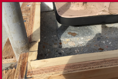
Setting Up the Forms
