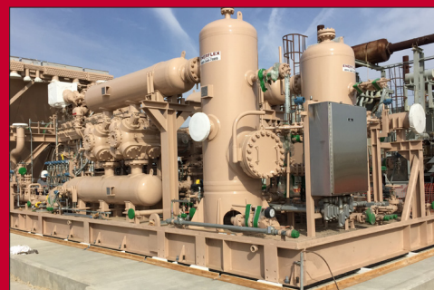
DP Epoxy Grout PG – Compressor Station Grouting
