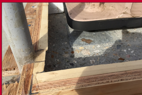
Setting Up the Forms
