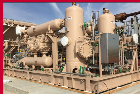
DP Epoxy Grout PG – Compressor Station Grouting
