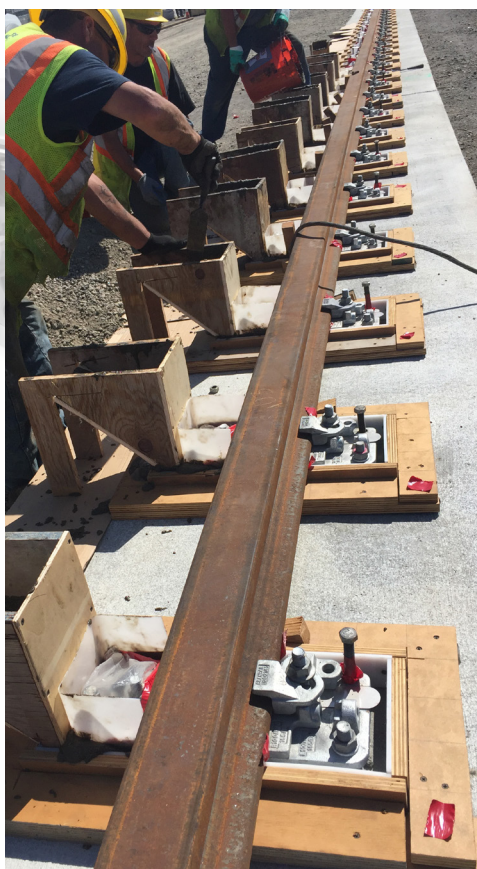
DP Epoxy Grout being used for crane rail grouting
