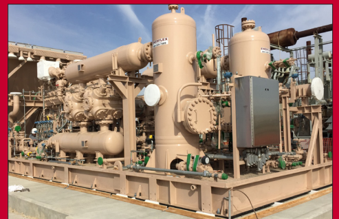
DP Epoxy Grout PG – Compressor Station Grouting
