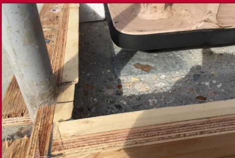
Setting up the forms
