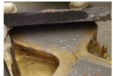
D.5. Screed off excess grout.
