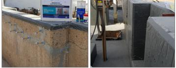
**The Challenge** — CalEnergy has been battling the effects of HCL in their containment pits for many years. They have tried numerous coatings that never lasted more than a few years at best. Concrete had eroded and crumbled. Steel reinforcement was exposed. Containment walls, sump pits, pump pedestals, containment floor and curbing were all compromised and in decline after years of failed protection.
