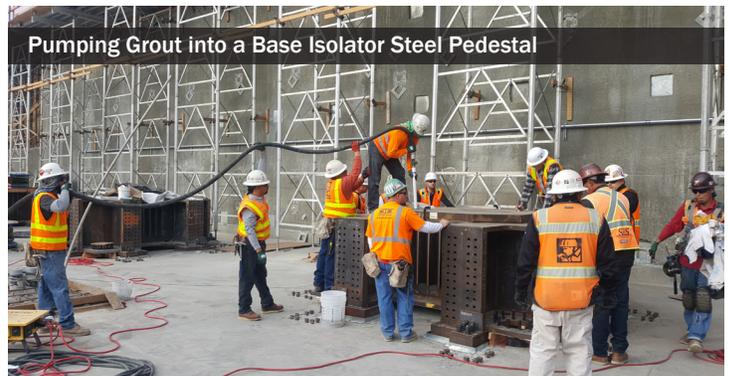
located in the center of the formwork the grout had to flow around. All of this combined with an increased minimum strength requirement of 13,000 psi and roughly 6 cubic feet of grout. Both joints required a 95% EBA minimum with no void larger than 1 square inch. Each joint would be disassembled and inspected for compliance throughout the duration of the project.
