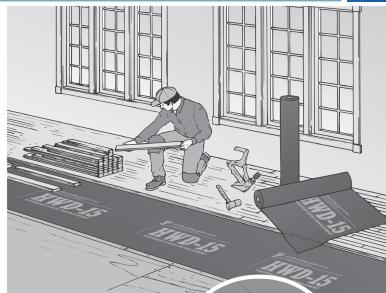
HWD-15 hardwood floor underlayment is an economical and extremely effective Class III moisture vapor retarder specifically designed for optimum performance in wood flooring applications. Consisting of a single layer of kraft paper saturated with asphalt, HWD-15 is a permeable vapor retarder. It reduces vapor flow, without trapping moisture.
