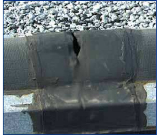
Splice Failure on Competitor's product
