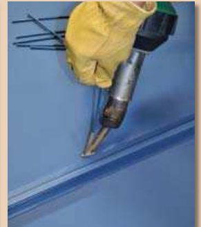
Step 5 - Permanently weld with SecureRod™
