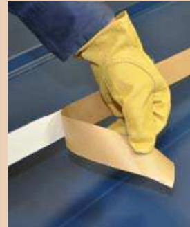
Step 4 - Remove tape/ affix to membrane
