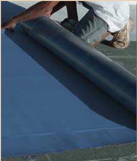
Step 1 - Install membrane
