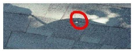
What Causes Fasteners/Nails installed on the face of the shingle... or below the fastening line results in Exposed Nails? exposed nails. When shingles are installed following GAF's application instructions, there will be no exposed nails in the field of the roof.
