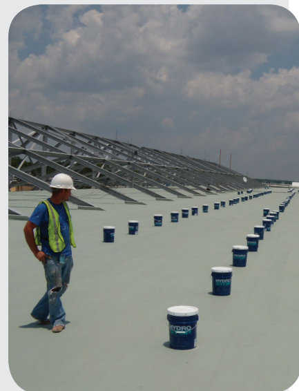
▲ National Guard Hangar - Jacksonville, FL
