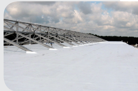
▲ National Guard Hangar - Jacksonville, FL
