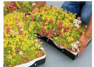
Certified Installer sets LiveRoof® modules tightly in place on the roof within RoofEdge® aluminum edge restraint.
