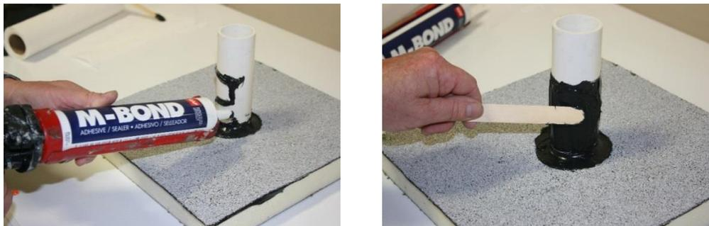
**Step #3-** Apply a bead of M-Bond around the entire bottom perimeter and an additional bead down the center. Apply a bead of M-Bond around the perimeter of the end joints. (Gray M-bond was used just to show the contrast on the black surface.)
