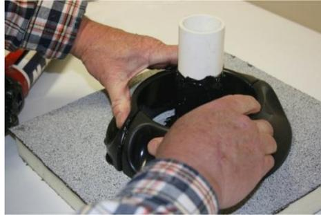
**Step #5-** Apply a bead of M-Bond around the outside base of the M-Curb and to the vertical joint sections. Tool the bead of M-Bond around the outside base and on the vertical joint sections.
