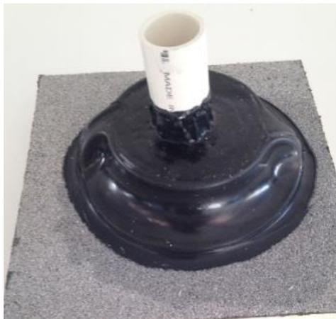
**NOTE:** A properly constructed M-Curb has four watertight seals; 1. M-Bond seal around penetration. 2. Pourable Sealer. 3. M-Bond seal under each M-Curb section. 4. Exterior perimeter M-Bond seal.
