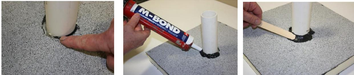
**Step #2-** Apply M-Bond to the vertical portion of the penetration and tool the sealant smooth. The M-Bond acts as a primer. The M-Bond shall extend up the penetration a minimum of 3". **DO NOT USE ASPHALT PRIMER OR ROOF CEMENT.**
