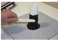
**Step #3**- Apply a bead of M-Bond around the entire bottom perimeter and an additional bead down the center. Apply a bead of M-Bond around the perimeter of the end joints. (Gray M-bond was used just to show the contrast on the black surface.)
