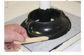
Step #6- and fill the entire M-Curb with M-Thane One-Part or Two-Part Pourable Sealant.
