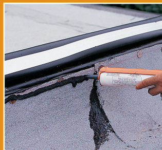
3 Apply Matrix™ 203 Plastic Roof Cement to vertical curb faces (or order with Metalastic® Butyl Tape Sealant), fold down and fasten outside nailer
