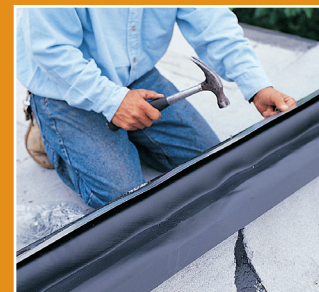
4 Compress bellows by aligning opposite nailing flanges with opposite curb edge and fasten
