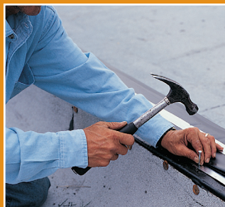
2 Nail inside metal nailer on one side
