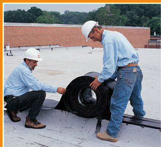
1 Unroll Metalastic® Expansion Joint Cover
