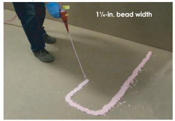
For Best Results: When applying adhesive, the end of the mix tip or the extension tube should be no more than 4- to 6-inches above the surface of the roof.
