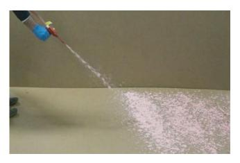
**Note**: Do not use the extension tube when using "spatter" technique. Pressurized canisters enable contractors to "spatter" the adhesive for use on fleece backed membrane. For best results, pull the trigger all the way to the handle and gently swing the gun back and forth while walking beside the
