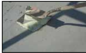
Fig. 4-3: Broken Bond
