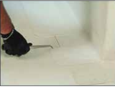
Fig. 4-8: Seam Probing
