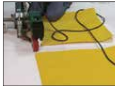
Fig. 4-11: Welding along non-textured ends
