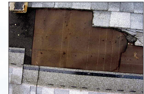
Blown-off shingles may expose your home to structural damage, mold, and mildew.
