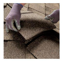
Place on the hip or ridge according to the exposure notch
