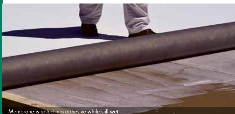
Membrane is rolled into adhesive while still wet
