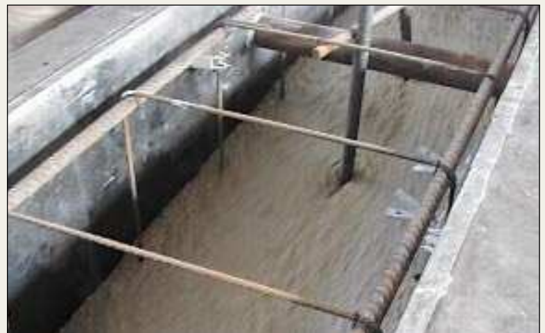
Self Consolidating Concrete in precast production fills formwork without segregation or blocking.
